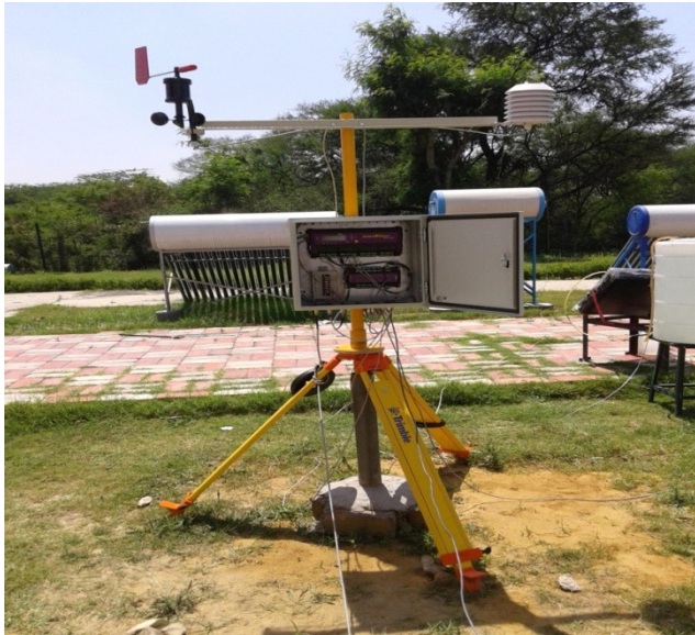
Fig. 2. Data Logger with Anemometer [NISE]
